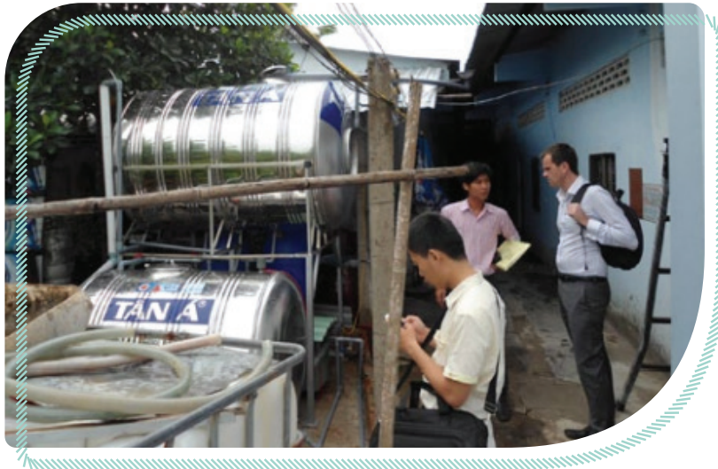
Figure 4: Rainwater Harvesting Systems in a Household in a Peri-Urban Area
